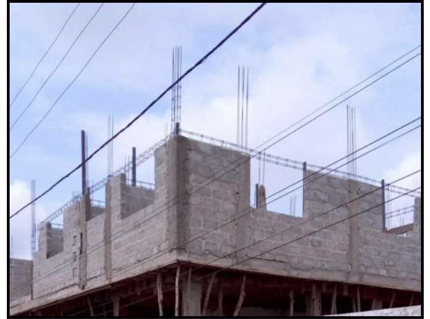
Calavi School Expansion Project
